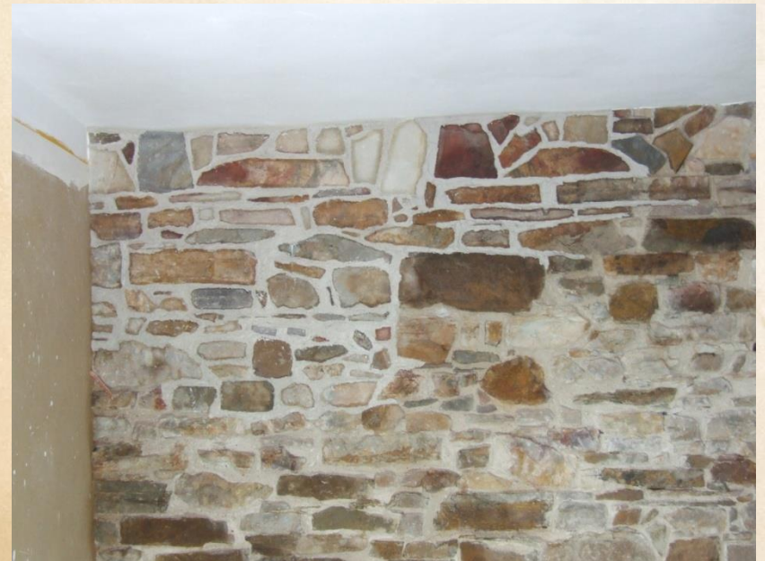
Back side of the stable wall – masonry work and joints
