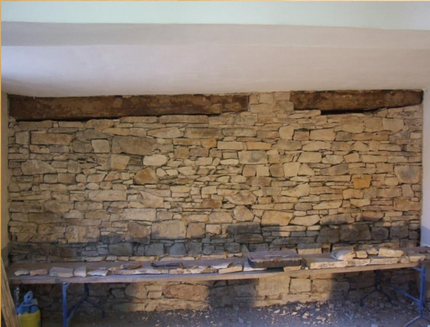
Back side of the stable wall – masonry work and joints
