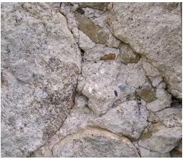
Figure 1: Historic hot-mixed mortar in a rubble wall, showing characteristic white lime inclusions
