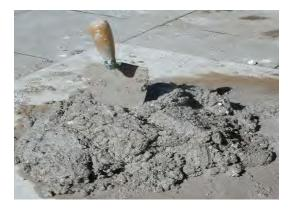
Figure 2: Sequence of photographs illustrating the hot-mixed mortar production method, covering quicklime with damp sand, allowing to slake and adding water to produce a mortar
