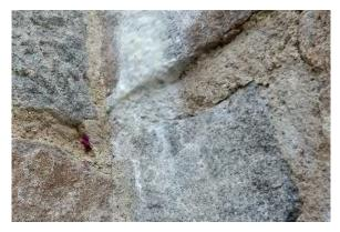
Figure 3: Leaching of mortar caused by Figure 3: Pitted harl finish caused by the poor building detailing and excessive wetting of masonry
