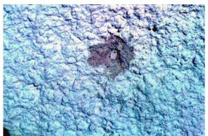
expansion of a particle of slow slaking quicklime after placing
