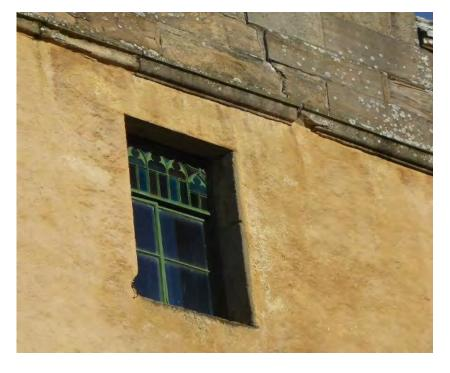
Figure 9.3 A close up of the upper part of the tower on the south elevation where a crack was observed below the chimney. Note the additional weathering below the open joint in the string course.
