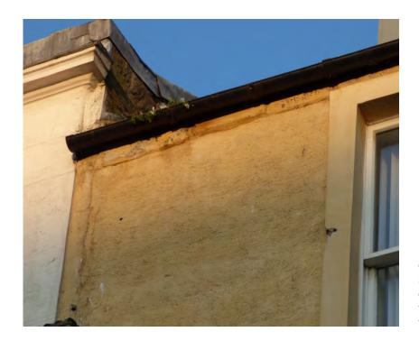
Figure 6.2 West side of elevation at roof level, showing some localised disruption of the harl from running water due to a blocked rhone.
