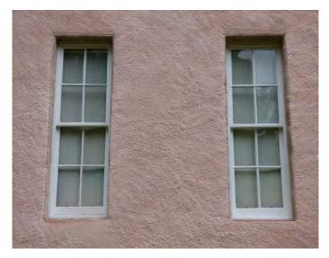
Figure 3.2 View of an area of wall, at first floor level on the west elevation, where the harl and limewash appear sound. No discolouration or erosion was detected at the cills, as is common below large windows where water sheds faster.
