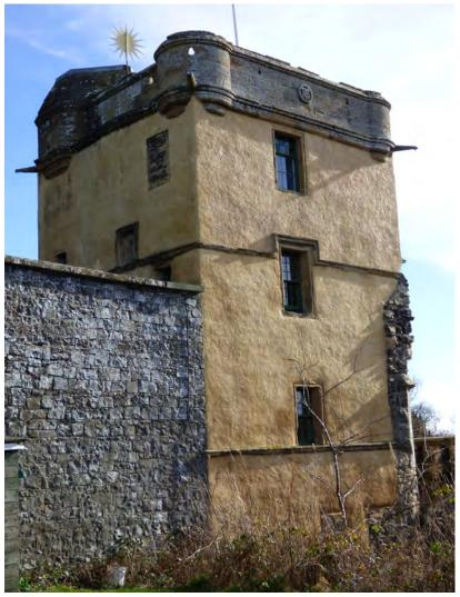
Figure 9.1 View of the west elevation of the tower, from the north-west, showing the slight colour variation in the limewash.
