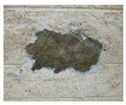
Figure 13.3 Close-up of one stone showing the mortar feathered over the edges of the stone, both effectively flattening the wall surface and displaying good adhesion to the masonry.
