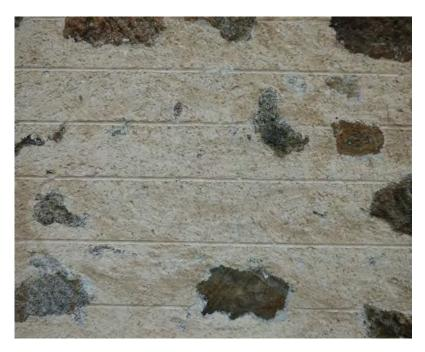
Figure 13.2 Close-up of an area of the pointing, showing a generally tight finish with a relatively uniform texture and finish.
