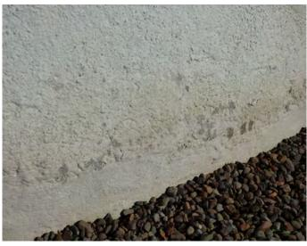
Figure 19.4 Localised spalling at low level in this area of repair.
