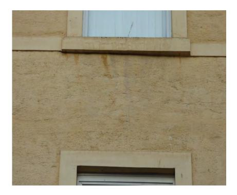
Figure 6.3 View of harl just above a first floor window, some faint horizontal cracking and discolouration of the limewash below the cill can be seen due to water draining over the cill.
