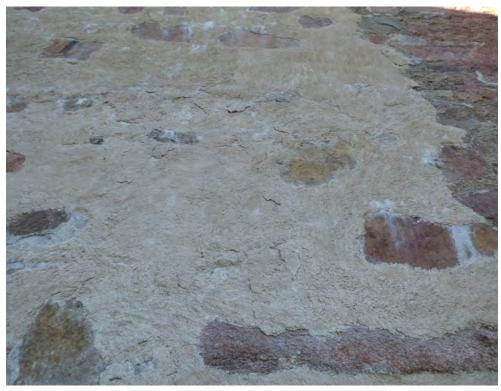
Figure 4.4 Section of pointing on the west wall, where scaling mortar and leaching of lime were observed. This example is directly below one of the parapet water spouts and adjacent to a large section of retained cement based pointing work.
