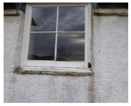
Figure 12.2 Window on the south elevation. The flaggy stone cill is deteriorating, as are all cills on this elevation, with a crack on the east side of window. Although there is evidence of channelled water flow over the cill, the underlying harl is sound and the limewash in relatively good condition.
