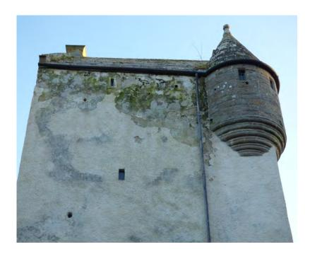
Figure 16.2 Extensive failure of the harling on the upper part of the northwest elevation, where there is total saturation of the wall head, probably due to poorly detailed rhones and a blocked downpipe.
