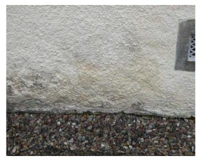
Figure 1.4 The harl at ground level on the rear elevation, showing some staining from rising damp, however, it remains well bonded.
