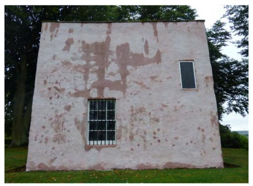
Figure 18.3 Rear (north) elevation, where the narrow overhang on the wall head cope is insufficient to keep water off the wall.
