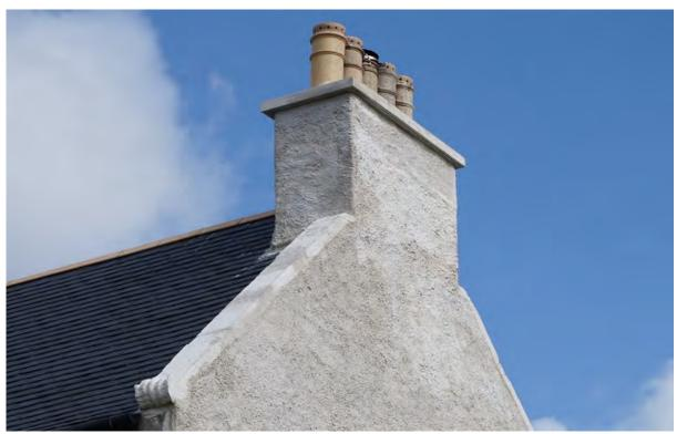
Figure 21.2 Detail of the chimney stack and upper gable, illustrating the harling and the limewash, the latter having been taken over the stone skews.
