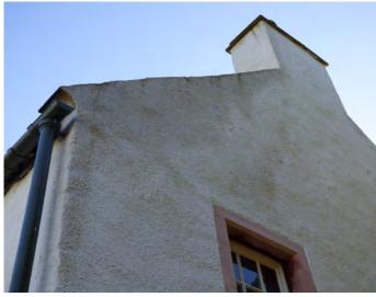
Figure 19.2 Evidence of rainwater wetting the wall below the north skew on the west gable, where water is running off the skew copes onto the gable.
