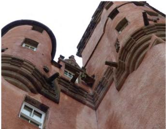
Figure 3.3 View of water spouts at third floor level all contributing to water discharge that is impacting on this corner at ground level.
