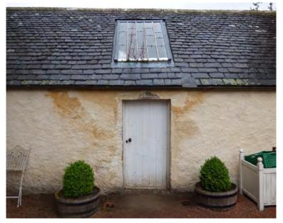
Figure 5.3 Rear elevation, with discolouration and some spalling from water damage. This is possibly caused by rainwater overtopping the gutters below the large rooflight.
