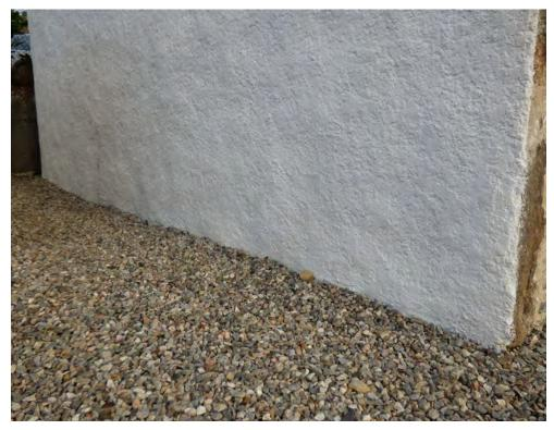
Figure 11.3 Base of the wall, showing harling carried on down to ground level.
