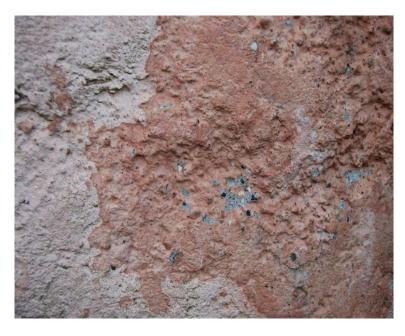
Figure 22.3 Detail of harling and limewash, with localised area of weathering/decay exposing underlying harl. The shell fragments can be seen in the harl finish.
