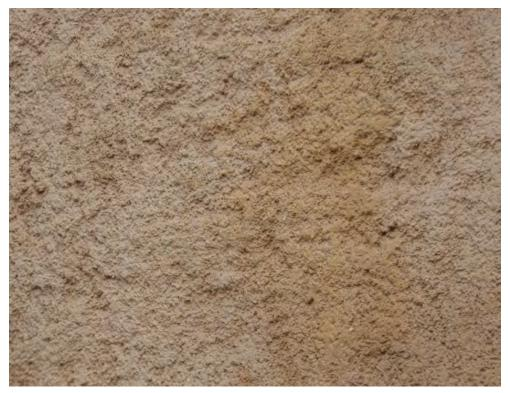
Figure 23.3 A close-up of the harl and limewash finish showing the aggregate distribution across its surface. The more open texture may be indicative of a mechanically applied harling.
