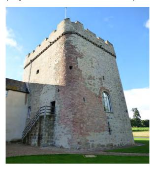
Figure 4.2 View of the south-west faces of the tower, affected by localised cracking and spalling of the mortar.
