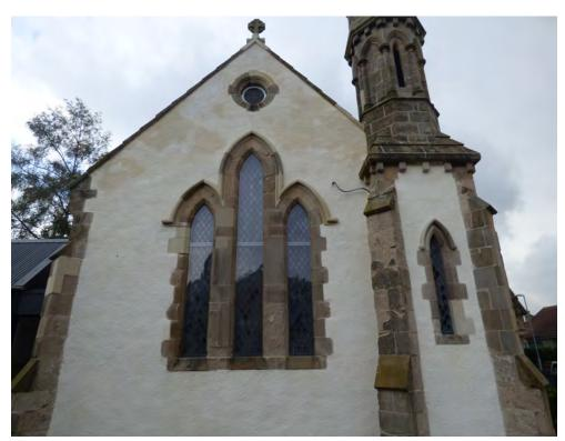
Figure 2.2 View of the west gable with bell tower. The harl and limewash are well finished and appear sound at this time. The limewash at upper levels shows the effect of wetting drying cycles.
