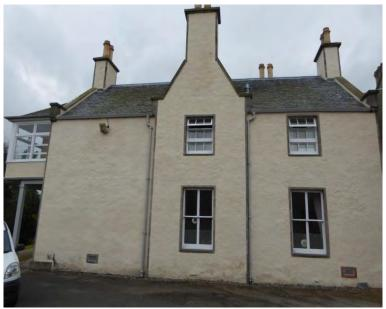
Figure 1.3 Rear elevation, the harl and limewash all sound, with the exception of rising damp and some mechanical damage at ground level.
