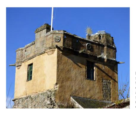
Figure 9.2 View of the south-east corner, with the localised area of disrupted harling apparent just below the string course on the north side of the east elevation.
