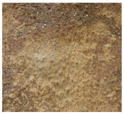
Figure 24.3 Close-up of an area of harl which has suffered from localised erosion, showing the range of limewash coats and the crushed shell.
