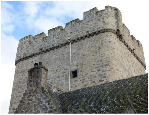
Figure 4.3 The east elevation of the tower, where the pointing appears to be performing well.
