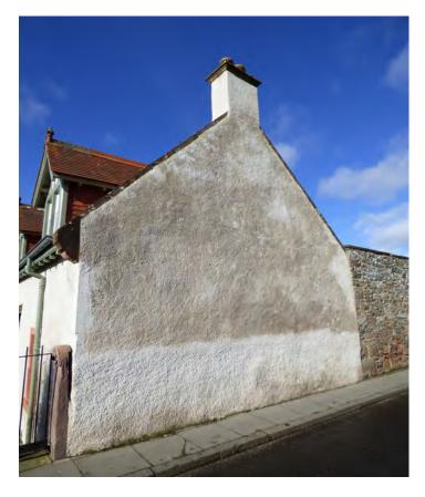
Figure 20.3 View of the east gable, showing the effects of a recent wall coating at lower levels.
