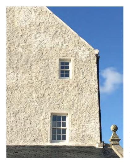
Figure 21.3 Detail of harling and limewash finish to southeast gable elevation, illustrating the textural effect of the harl in direct sunlight and the colour variation due to wetting and drying.
