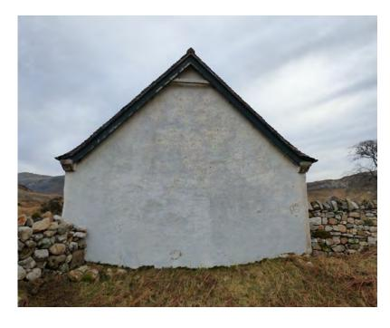
Figure 12.3 The lime harling on the very exposed west gable remains in good condition. There is some loss of limewash, which is to be expected due to the exposed nature of the site.
