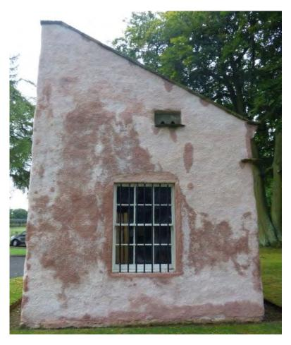
Figure 18.2 View of the west gable, showing extensive discolouration. This is mostly due to insufficient overhang on the skew cope above, and wind driven rain having recently played on the surface.
