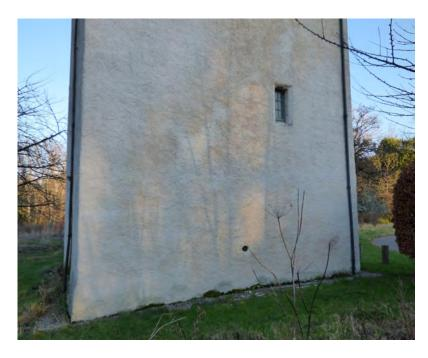
Figure 16.3 Base of the south-west elevation showing the harling and limewash to be in good condition.
