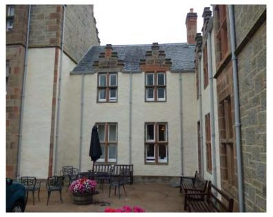
Figure 1.2. Harling to the front elevation, east side of the tower. The harl and limewash all appear to be uniform and in a sound condition.
