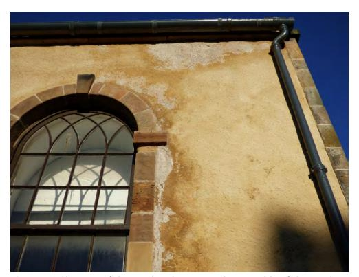
Figure 7.4 Close-up of the erosion damage at the east side of the south elevation, caused by blocked or poorly configured rainwater goods above, now rectified.
