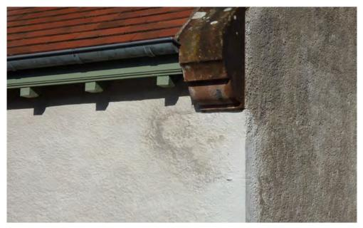
Figure 20.2 View of the skew putt on the south-east corner, which shows some minor staining of the limewash due to water run-off from the skew putt.
