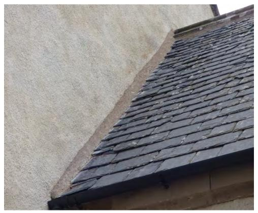
Figure 2.3 Slight patchiness was observed on the east gable, which is not uncommon in limewashed harl, particularly following periods of rainfall and subsequent drying.
