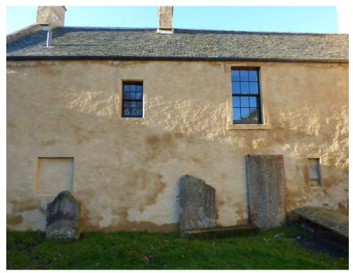
Figure 7.3 East elevation, which is generally in a sound condition, with localised discolouration of the harl, again due to both rising and draining dampness and the drying of the wall fabric below.
