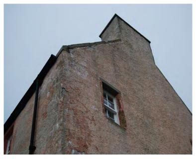
Figure 22.2 South-west corner illustrating a number of defects to the harling; cracking and localised detachment of harl, localised lime leaching and partial loss of limewash.
