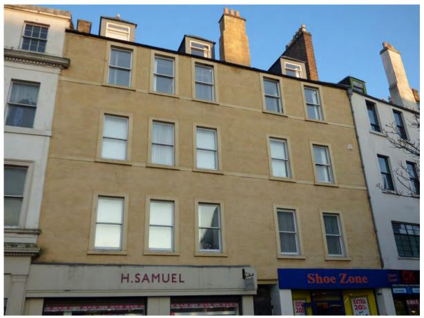
Figure 6.1 Front elevation showing the generally good condition of the harling.
