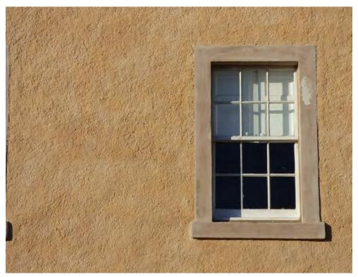
Figure 8.2 View of an area of harl, to the west of the easternmost window, at first floor level. Here the subtly undulating profile and texture of the harl can be seen to be enhanced by the warmth of the limewash coating.
