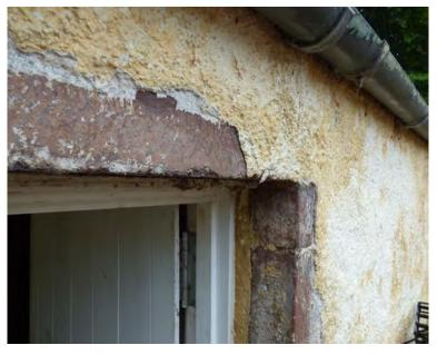
Figure 5.4 Loss of harl from the lintel and the sandstone dressings to the ingo at the east doorway on the front elevation.
