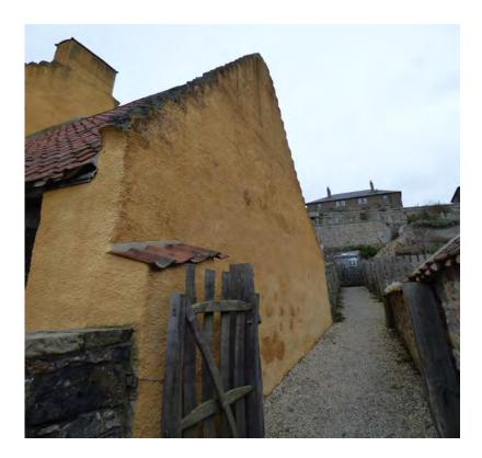
Figure 10.2 View of the east gable of the east extension. Staining at the crow steps is clear, as is blotching from salts within the wall lower down.
