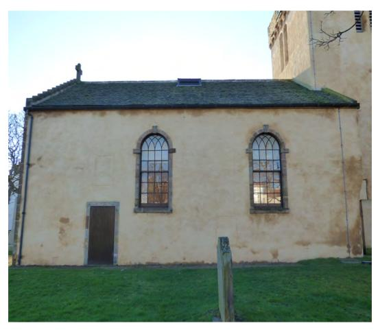
Figure 7.2 North elevation, where the harl appears sound and well bonded. Localised discolouration seems to be due to water run-off and from drying of the previously saturated walls.
