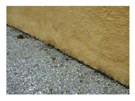
Figure 10.3 View of harl close to ground level. The harl has been terminated just above ground level to minimise wicking.
