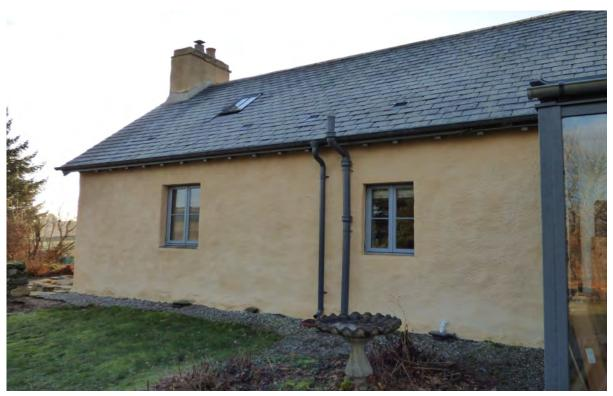
Figure 14.2 North elevation, west side. The harling is slightly textured and undulating following, to some degree, the profile of the masonry.
