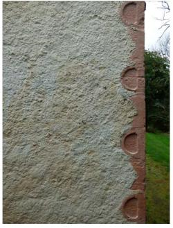
Figure 15.3. The east corner showing the well feathered junction with the sandstone quoins.
