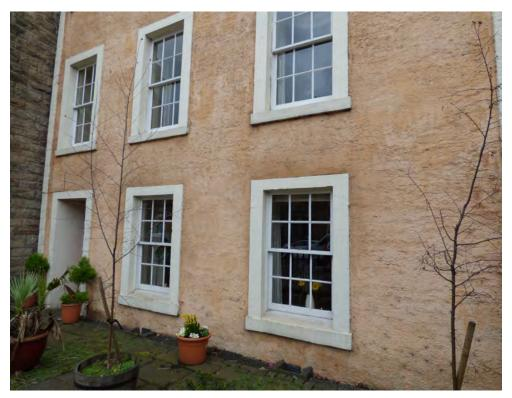
Figure 23.2 General view of the ground floor elevation, showing intact harl.
