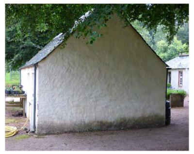
Figure 5.2 West gable, with the limewash and harling over most of the wall area in good condition. The exception is at ground level which is marked by soiling and wetting due to long term splash back from rainwater dripping from the roof.
