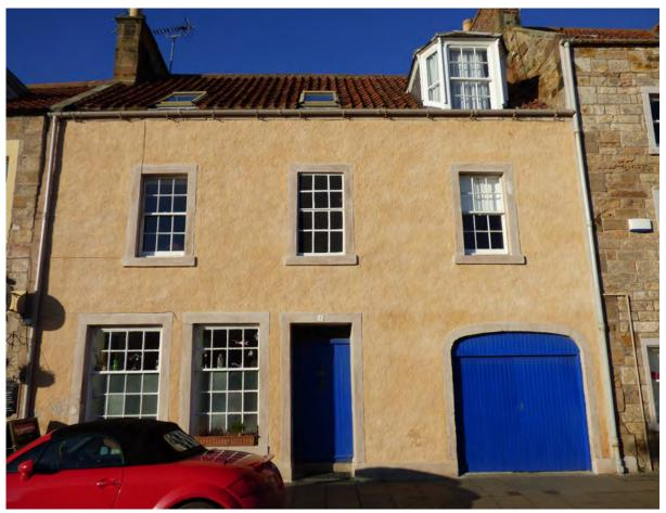
Figure 8.1 Front (south-east) elevation, showing the uniform appearance of the limewashed harl over the full elevation.
