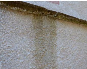
Figure 19.3 Staining of the harl of the stepped extension on the west gable, where the drip detailing is damaged or insufficient.
