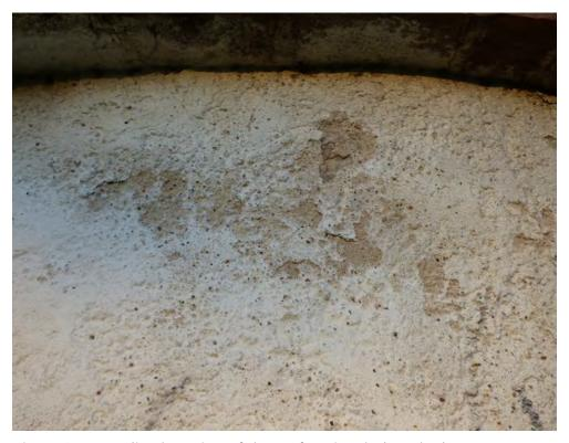
Figure 17.3 Localised erosion of the surface just below the lower stone rat ledge on the west side.
