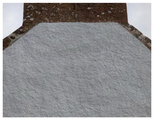
Figure 11.2 Close-up of the harling termination at the chimney.
