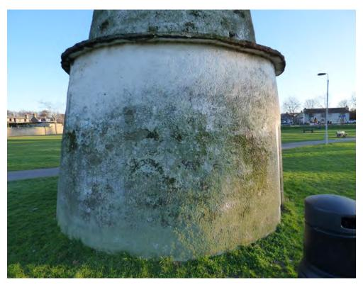
Figure 17.2 North side of the doocot showing the generally sound condition of the harl.
