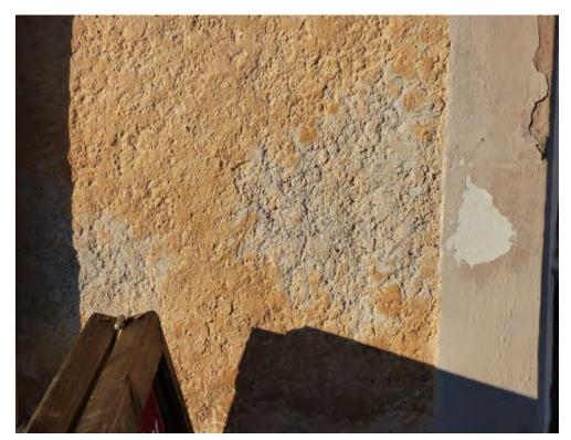
Figure 8.3. West side of the facade, at low level, where damage to the surface is evident. There has also been localised loss of the finish coat and limewash to the window dressing of the westernmost window.
