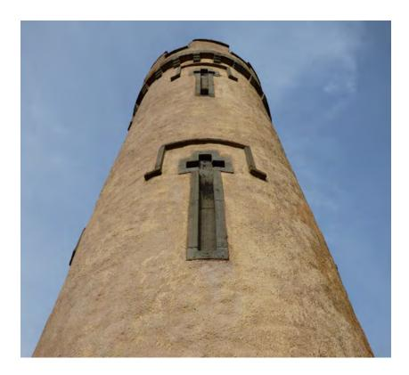
Figure 24.2 View of the upper part of the east elevation showing the weathering and the discolouration of the limewash on the north (right) side of the tower. This side has the most colour variation.
