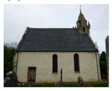
Figure 15.2 South elevation, showing the staining from water run-off below the cills and the damage from the overflowing of the rhones at the wall head.
